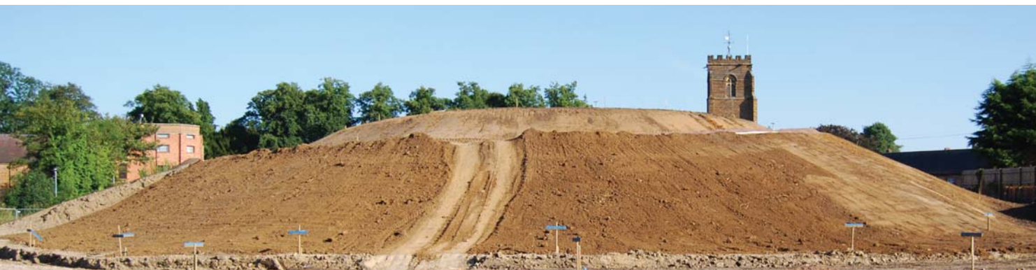
Bury Mount restoration in progress, 2009
